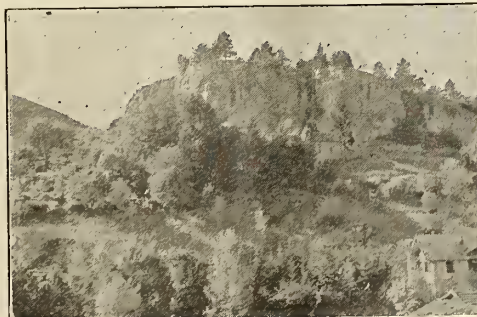
THE VIEW FROM THE REAR OF THE BUILDING WHERE THE MEN LIVE.
